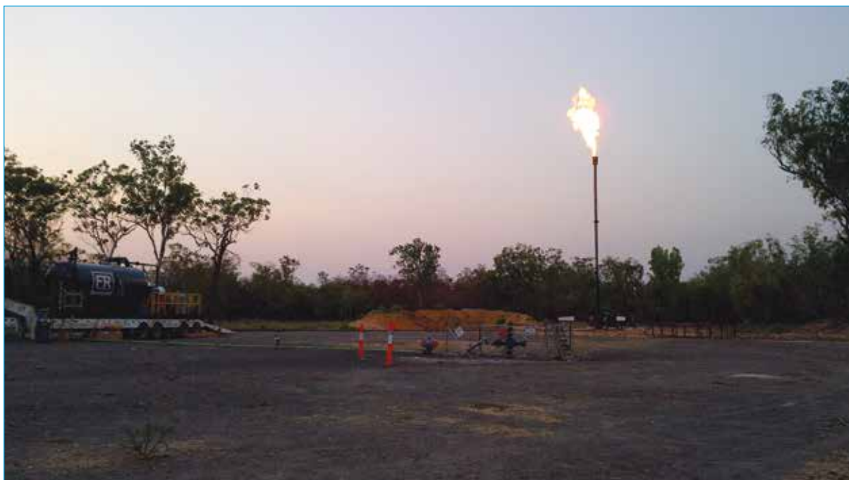
Production testing at Waggon Creek-1.
